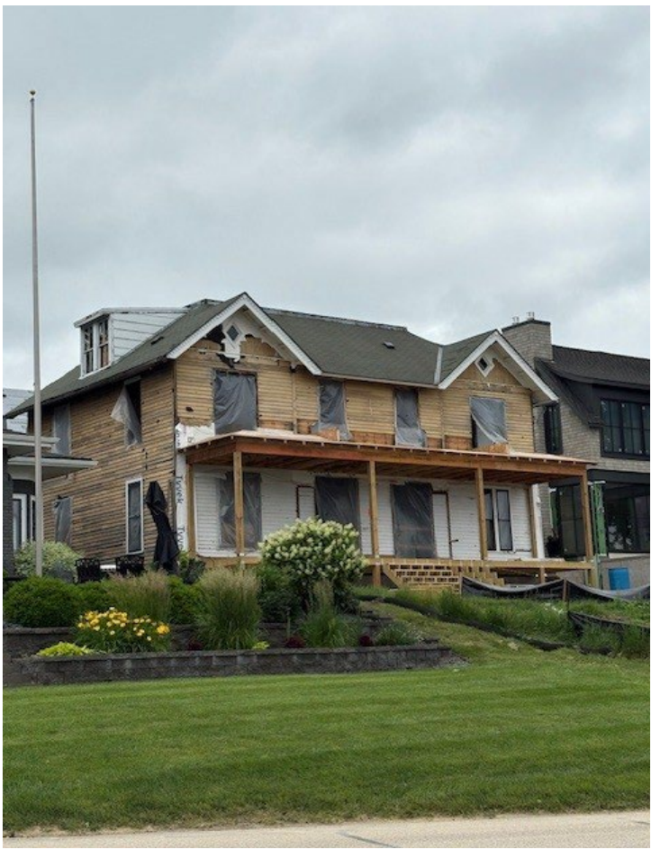
FRONT PORCH VIEW
