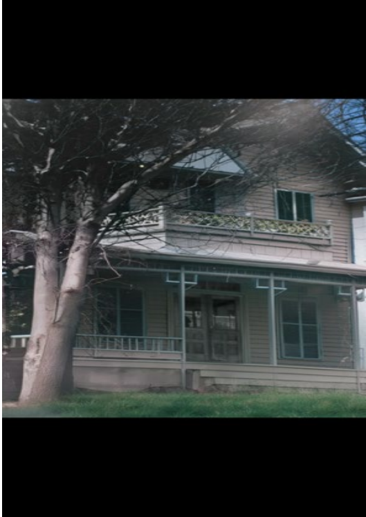
ORIGINAL PORCH WITH DECK
