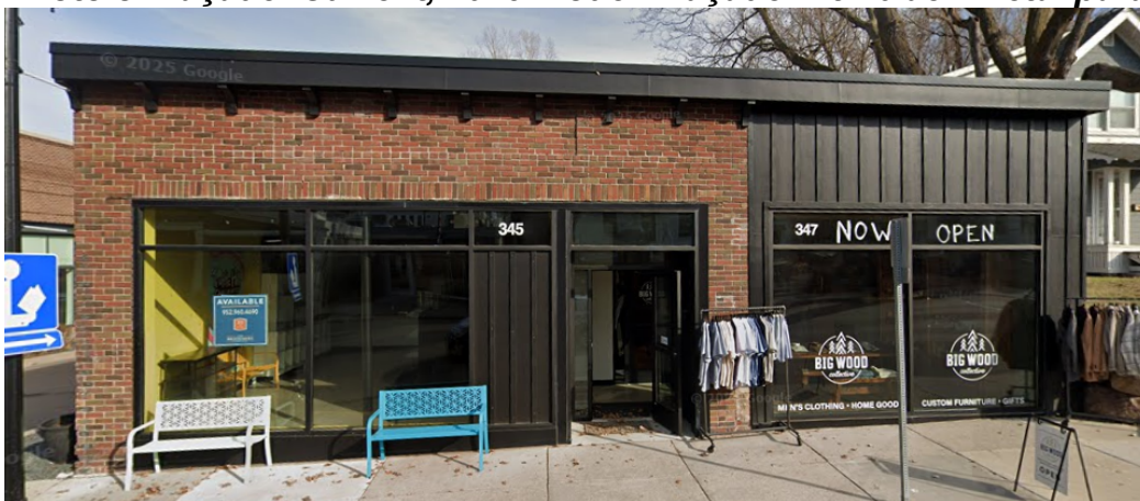
Photo of Façade: Current, 2025 modern façade with black metal parapet.
