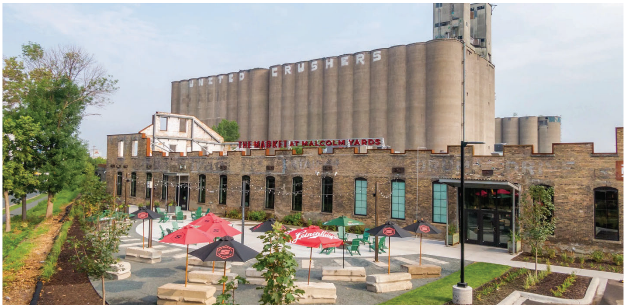
Malcolm Yards Market – AFTER Construction
