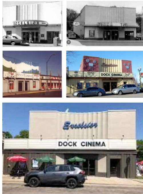
Fig. 5. Tonka Theater, façade, from SAP application.
