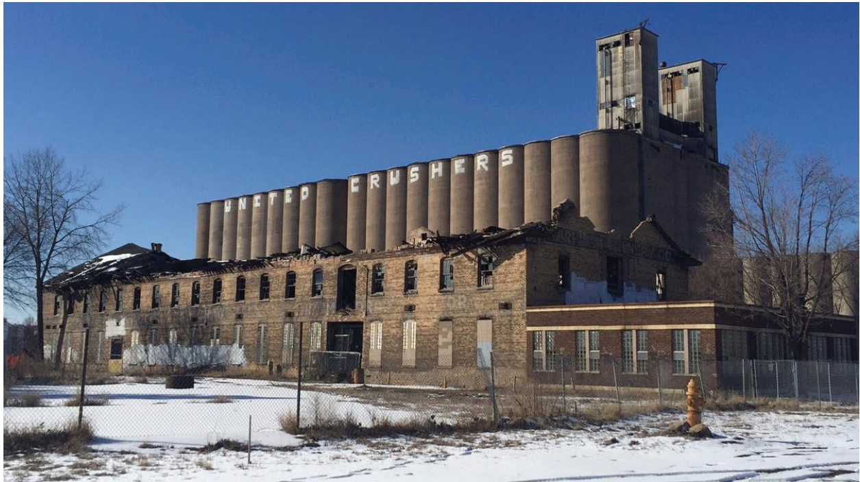
Malcolm Yards Market – BEFORE Construction
