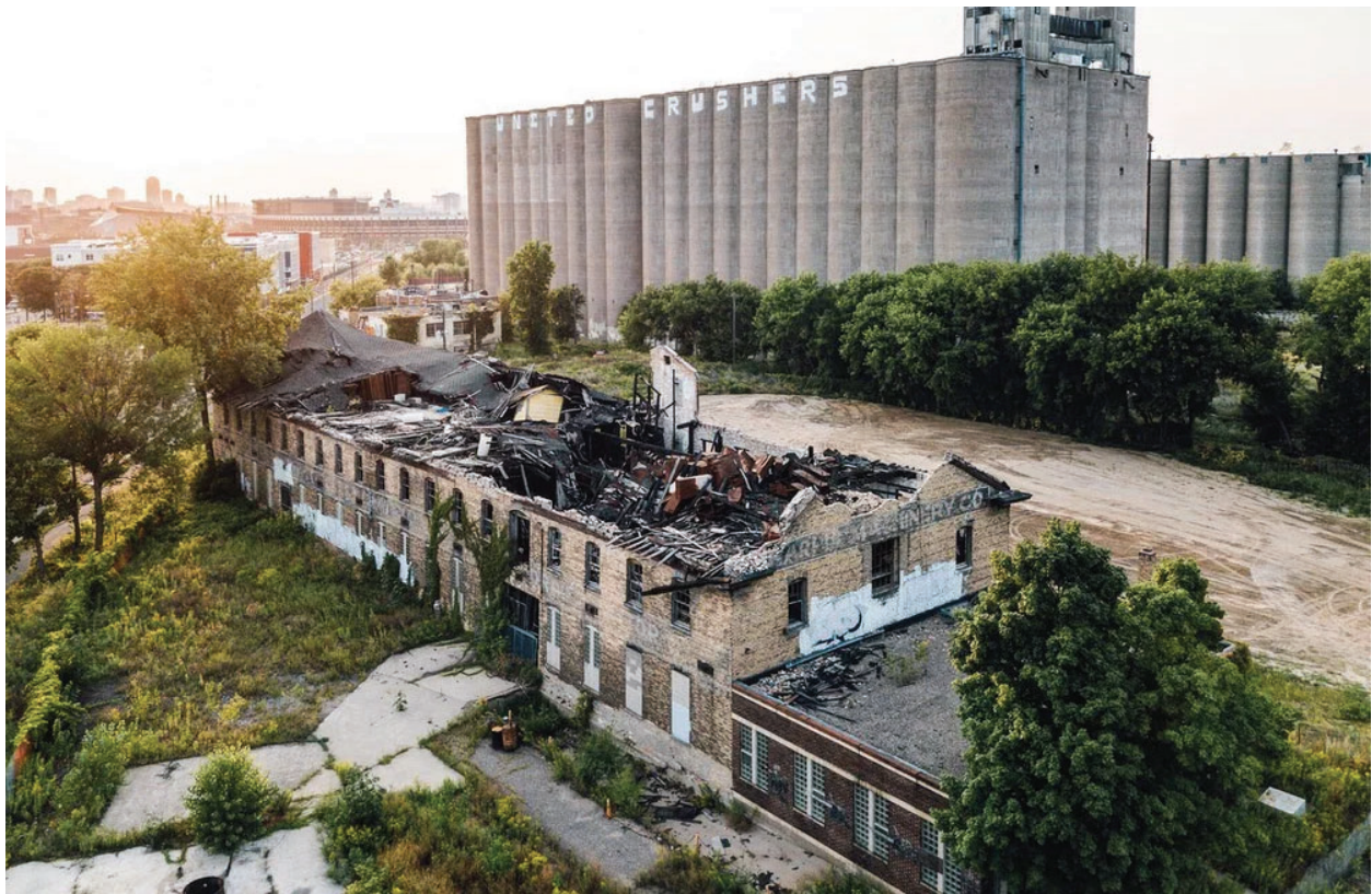
Malcolm Yards Market – BEFORE Construction
