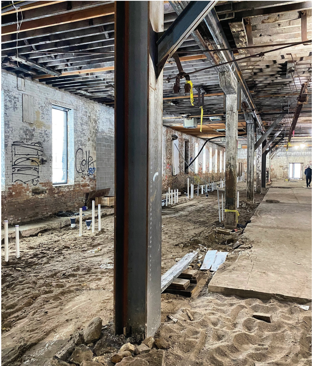
Malcolm Yards Market – DURING Construction
