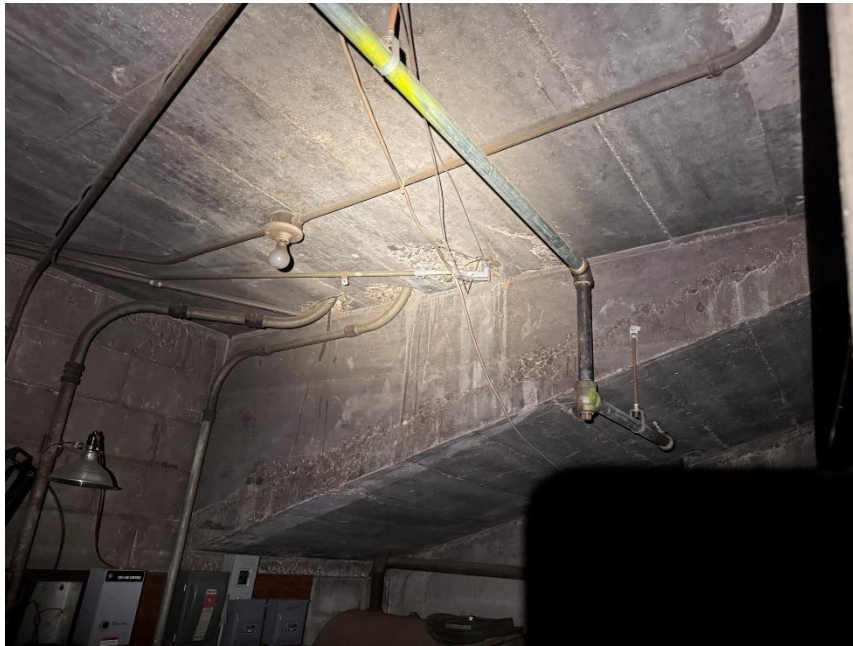
Figure 2: Concrete construction at steep egress ramp
