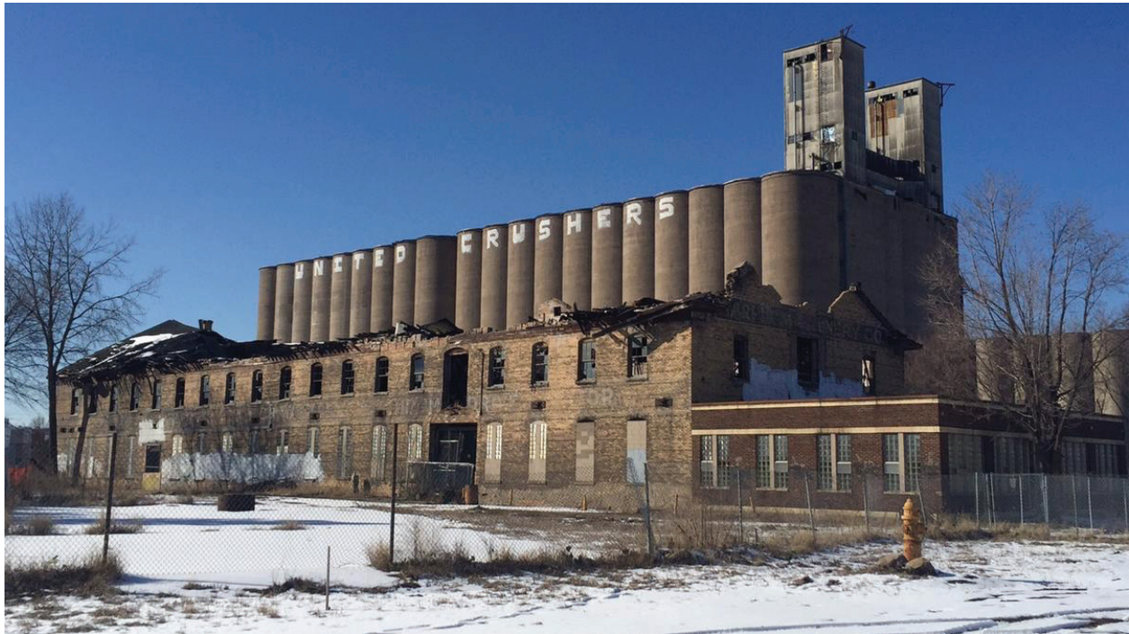
Malcolm Yards Market – BEFORE Construction
