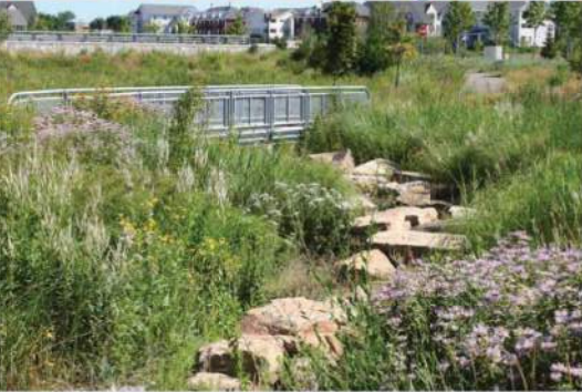
green stormwater infrastructure
