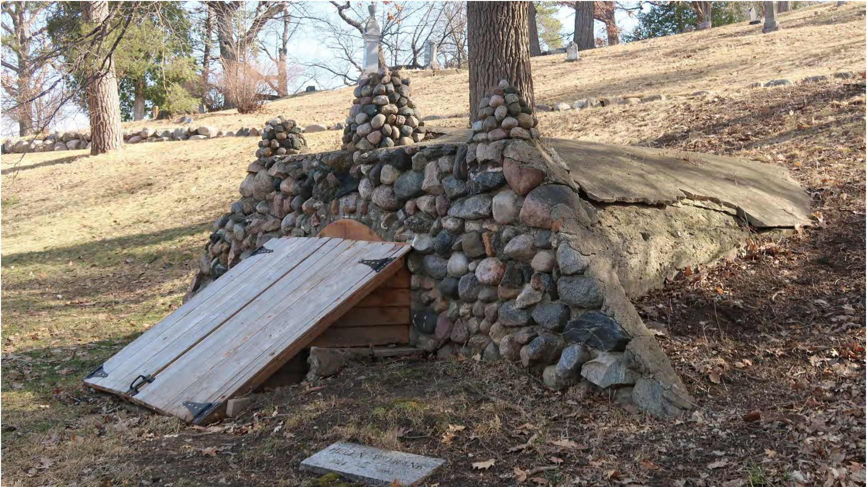
Figure 6: Vault at Oak Hill Cemetery, Excelsior. Vie to northeast. March 2026.
