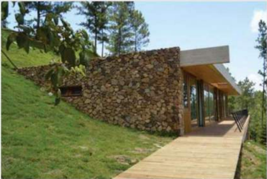
restroom + watercraft rental building built into the hillside
