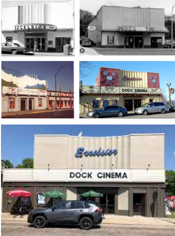
Fig. 4 Tonka Theater, façade
