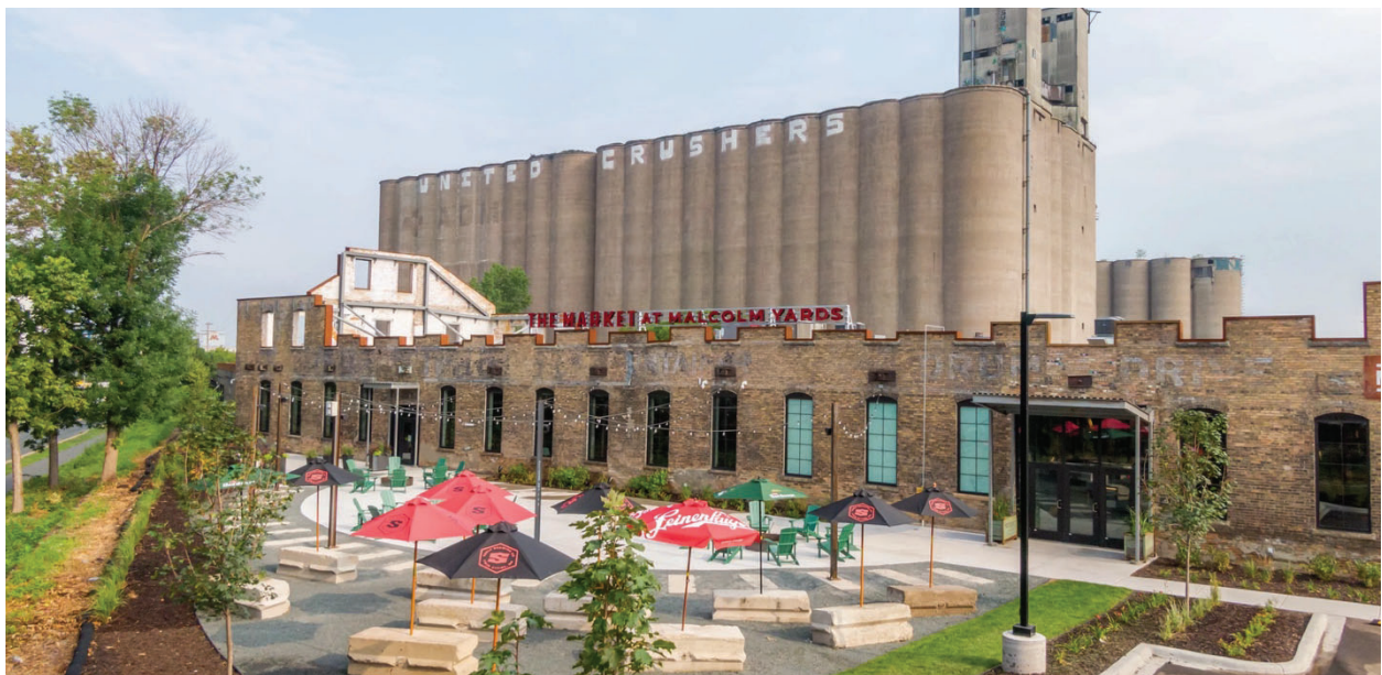
Malcolm Yards Market – AFTER Construction
