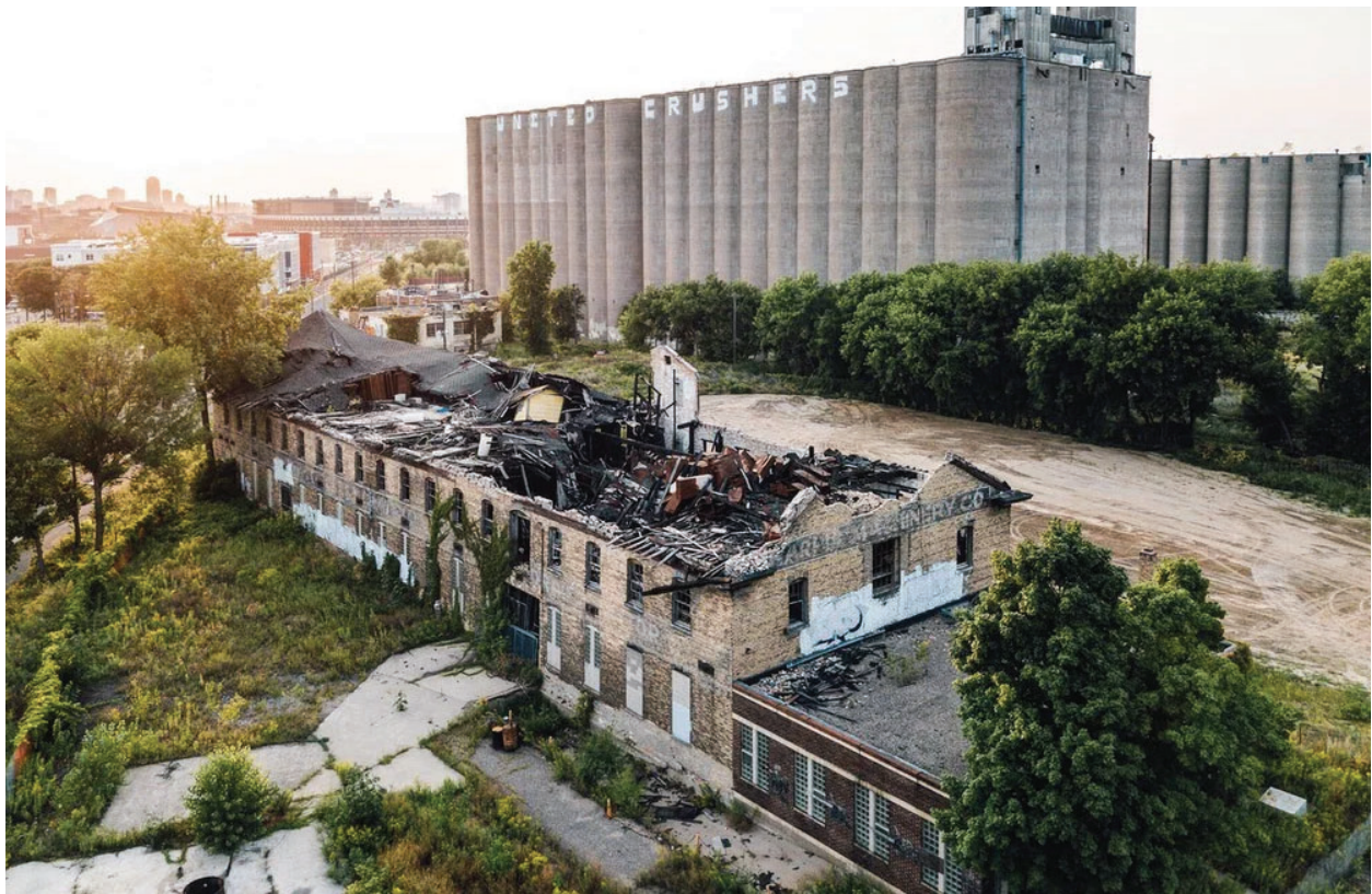
Malcolm Yards Market – BEFORE Construction
