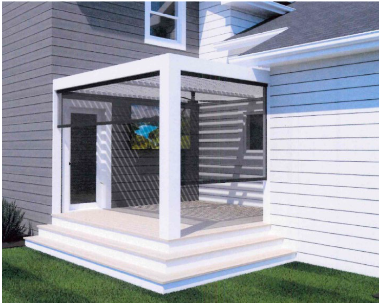
Figure 1 Example of rear porch with slatted roof and screens
