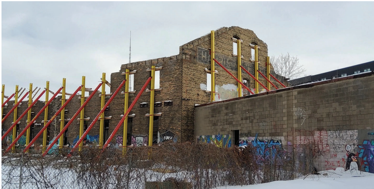
Malcolm Yards Market – DURING Construction
