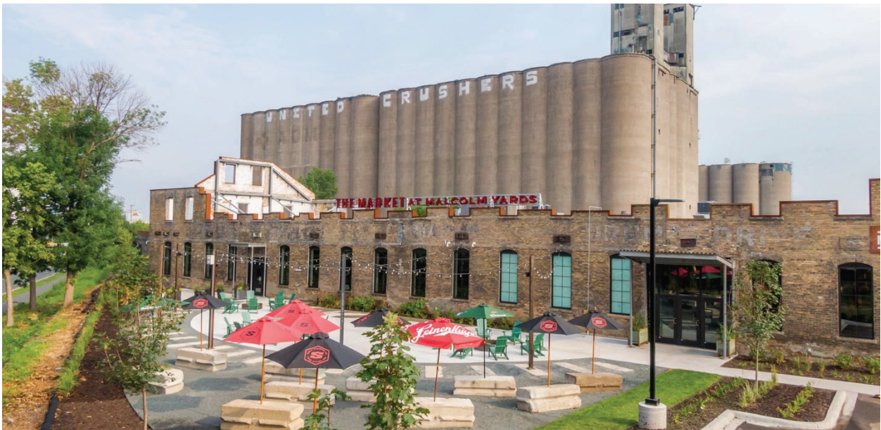
Malcolm Yards Market – AFTER Construction
