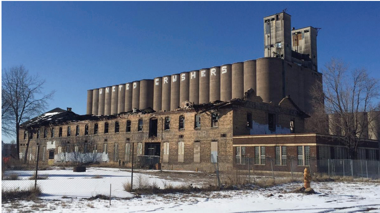
Malcolm Yards Market – BEFORE Construction
