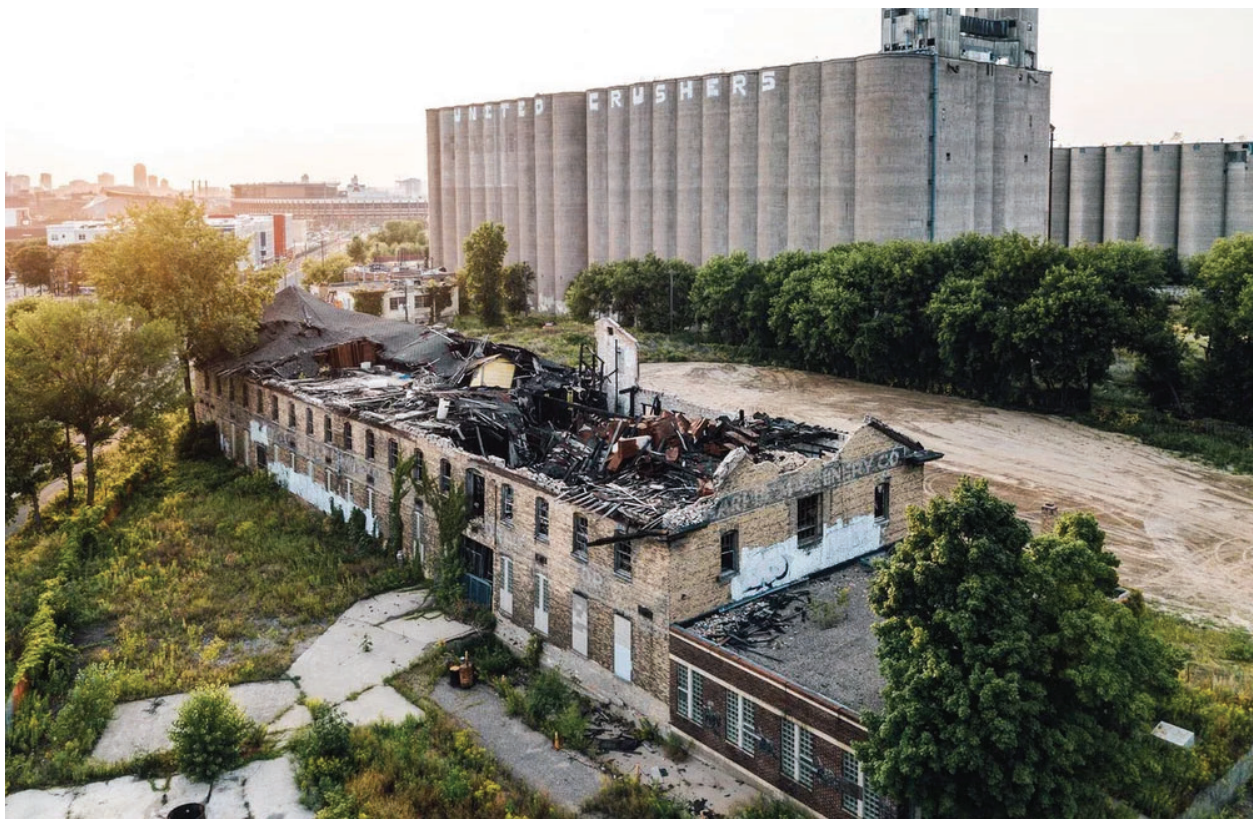
Malcolm Yards Market – BEFORE Construction
