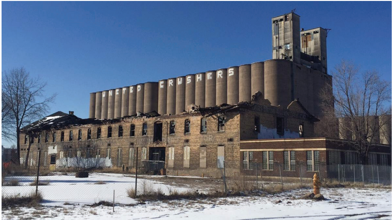
Malcolm Yards Market – BEFORE Construction
