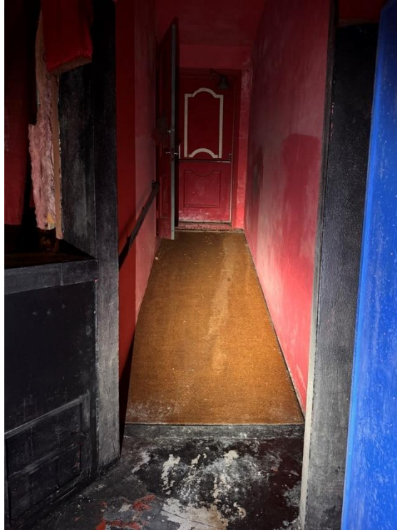
Figure 1: Narrow and steep concrete slab at egress
