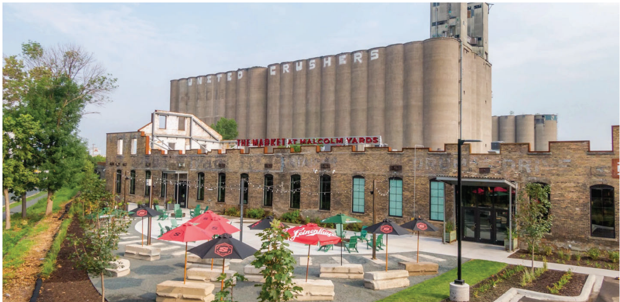
Malcolm Yards Market – AFTER Construction
