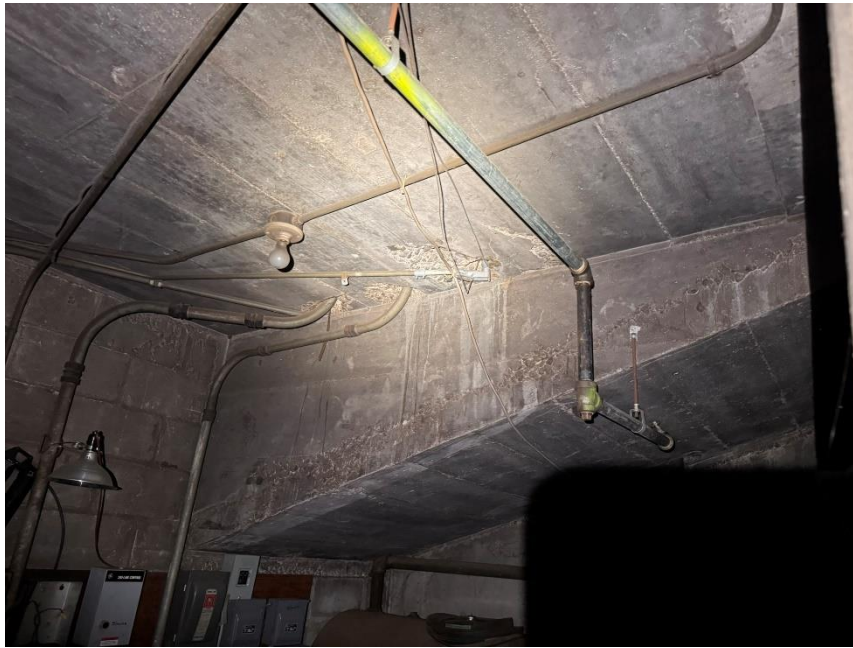
Figure 2: Concrete construction at steep egress ramp
