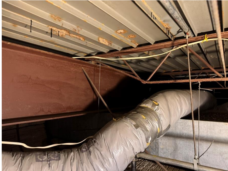
Figure 3: Steel roof framing (not at roof leak area)
