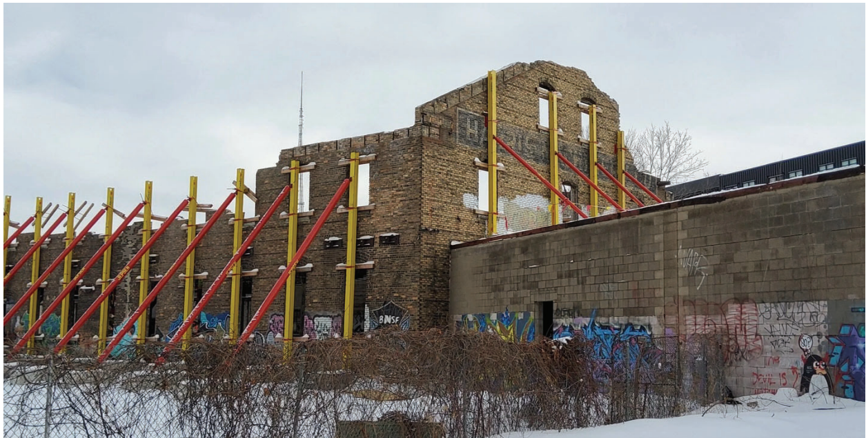
Malcolm Yards Market – DURING Construction
